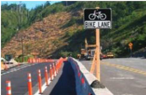
In general, no signs are required for shared roadways. However, they are installed for safety reasons to inform roadway users that bicyclists can be expected in the travel lane and near intersections. They might be placed near construction zones where bike lanes are temporarily blocked.
