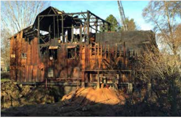
Butte Creek Mill before restoration.
