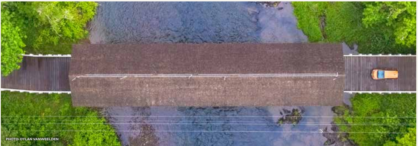
Oregon Electric Byways, EV at Pengra Covered Bridge outside Jasper.
