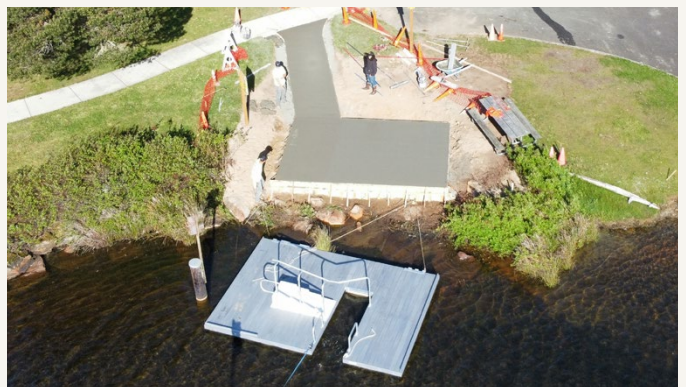
The cement and launch have been installed at the first ADA kayak launch on the Southern Oregon Coast as part of the Tugman State Park project. Photo Credit: Ollie Koerber/ Brock Concrete
